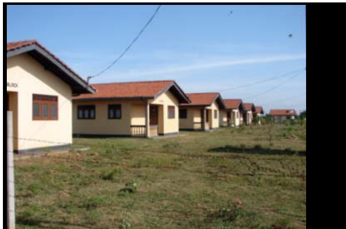
An abandoned relocation site in Hambantota district. Due to lack of services and distance from employment opportunities tsunami-affected communities refused to relocate
