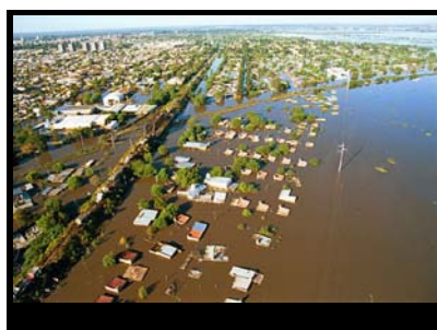
The Salado River which is exposing the city of Santa Fe to the risk of floods
