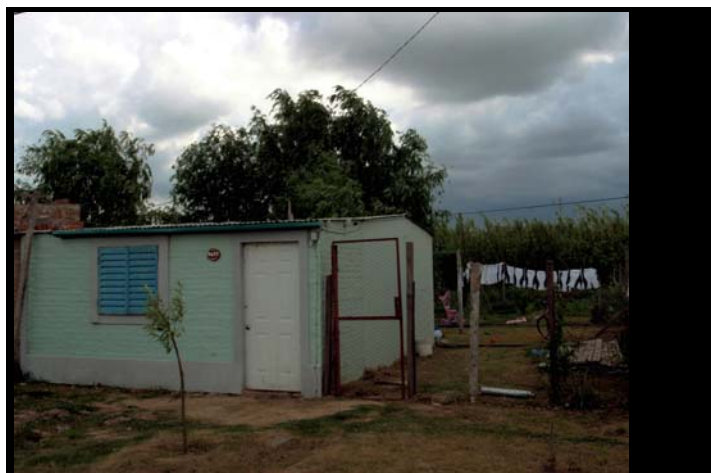
A plastic house provided within the framework of a resettlement project after the floods of 2003
