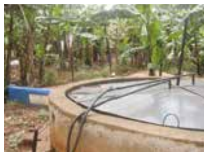
Photo about a rural biogas plant using agricultural waste for biogas production and nutrients recycling
